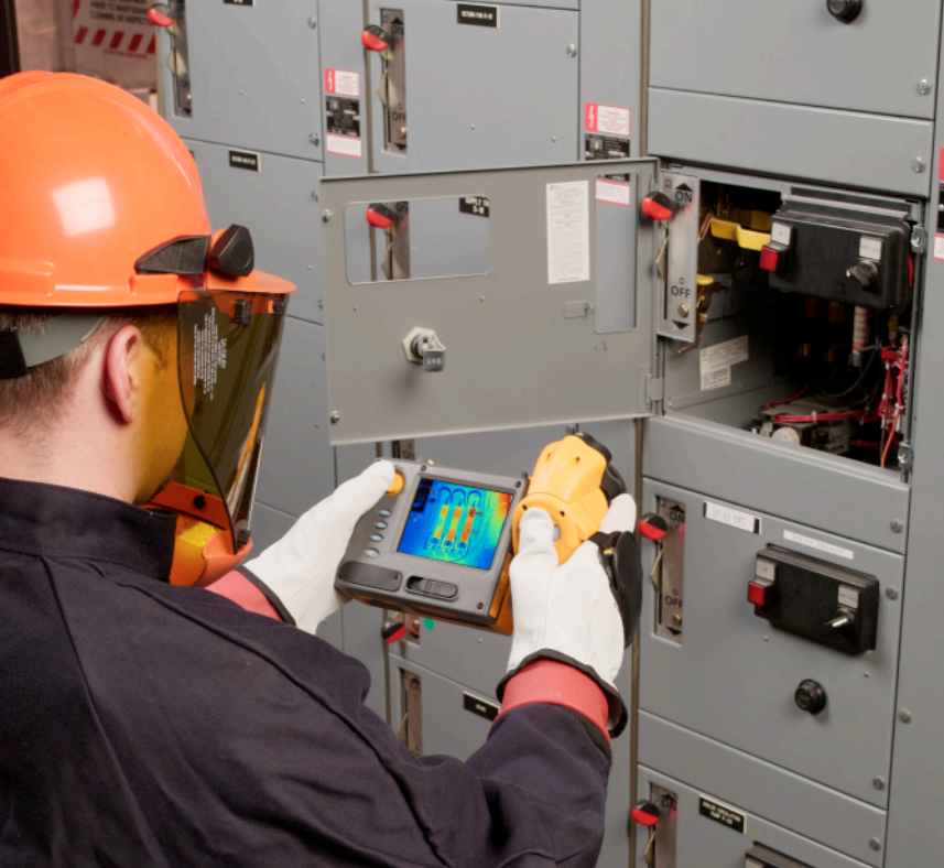
A thermal imager can uncover problems that might cause inefficient energy consumption.
