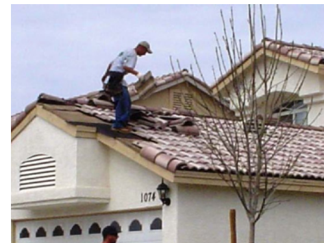
Expert performing testing on residential roofs.
